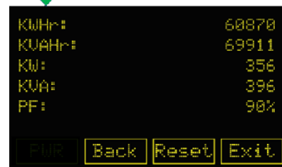
Power Metering Screen
